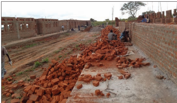
Construction of boy's dormitory in progress.
